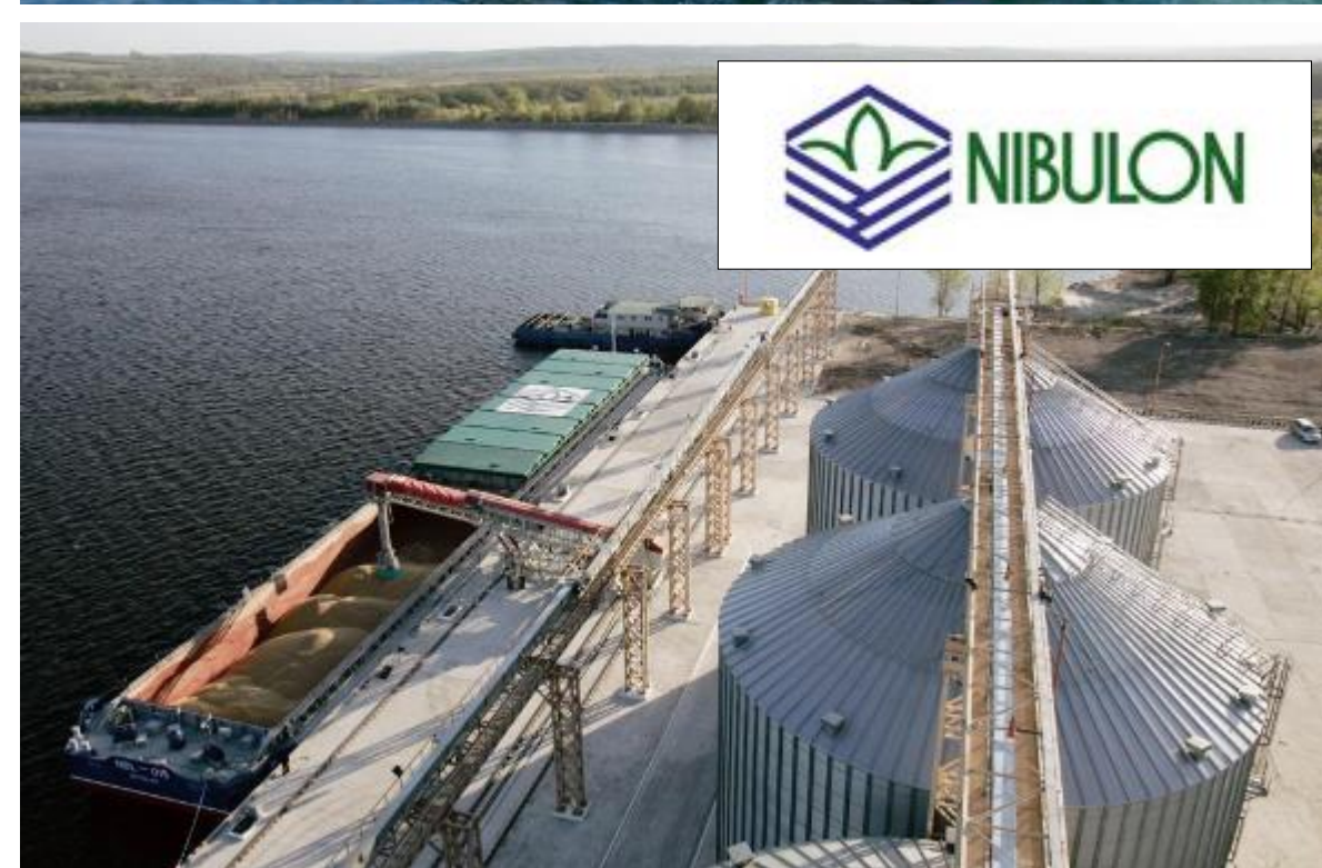
4 x discharge points from conveyor system onto Mobile Shiploader
